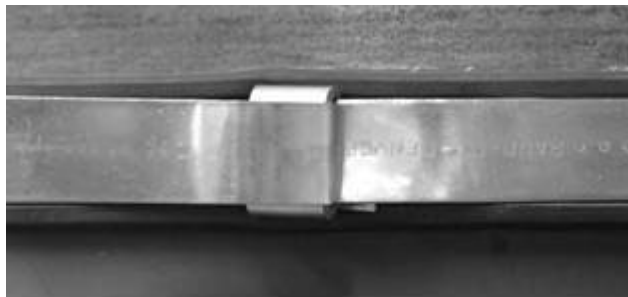
Figure 2-20: Band Clamp Final Installation
