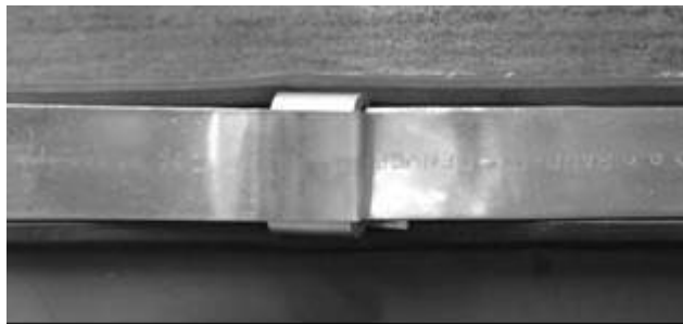
Figure 2-20: Band Clamp Final Installation
