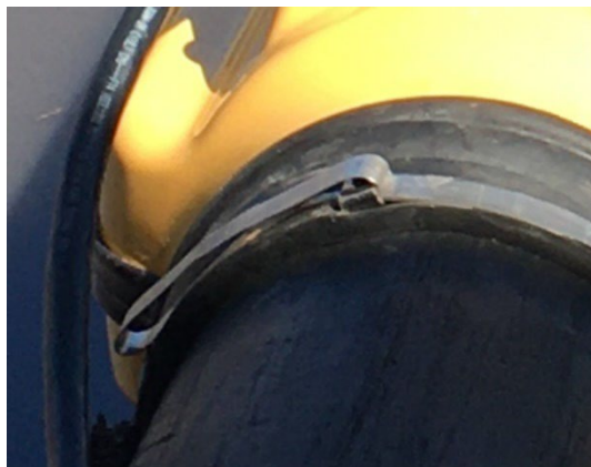
Figure 2-21: Alternative Band Clamp Final Installation
