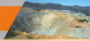
The Mine Complex uses conventional open-pit mining methods including drilling, blasting, loading, hauling, and crushing.
