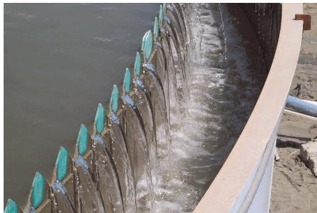
Figure 10 Clear Water Exit Channel
