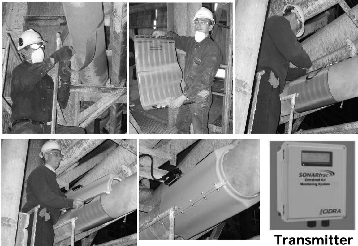
**Figure 7** Installation procedure from (top-left) pipe preparation through cleaning and light sanding of pipe to (top-middle and top-right) mounting of the flexible, lightweight sensor band to (bottom-left) installation of this sensor cover and to (bottom-middle and bottom-right) connection of sensor cover to transmitter via water tight cable
