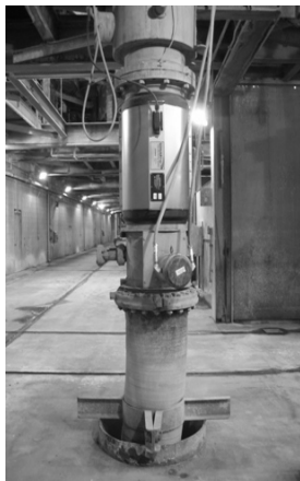
Figure 8 Sonar Based Flowmeter Exhibits Lifetime > Pipe
