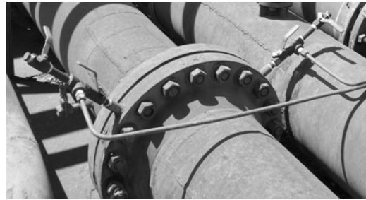
Figure 5 Invasive Orifice Plate Flowmeter with Pressure Taps
