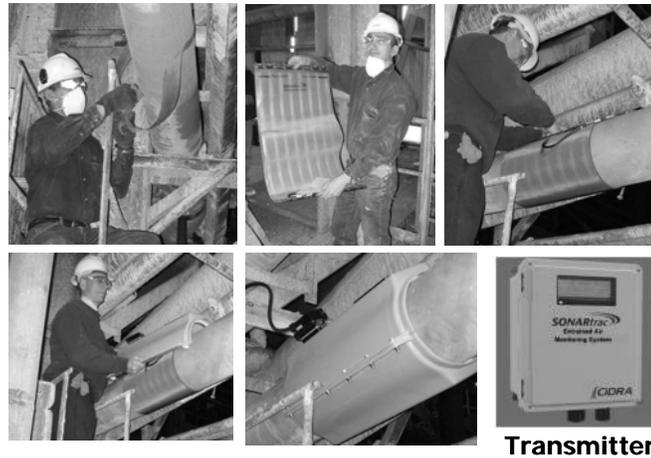
**Figure 5: Installation procedure from (top-left) pipe preparation through cleaning and light sanding of pipe to (top-middle and top-right) mounting of the flexible, lightweight sensor band to (bottom-left) installation of the sensor cover and to (bottom-middle and bottom-right) connection of sensor cover to transmitter via water tight cable**
