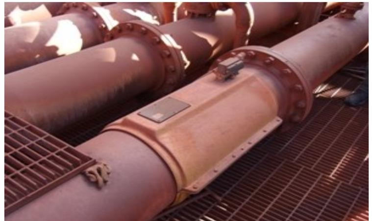
*SONARtrac* Process Measurement Systems, sonar-based clamp-on technology for the most challenging processes.
