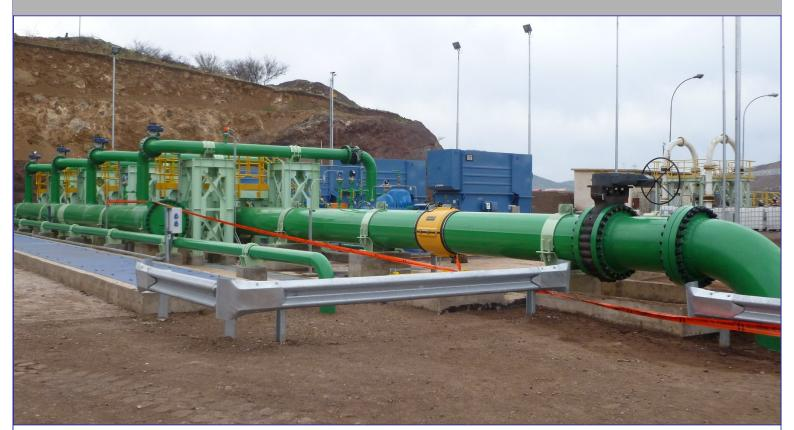
CiDRA has exceptional field experience with water applications, particularly where scale build up is an issue. The *SONARtrac* clamp-on system provides a non-intrusive, reliable measurement of the volumetric flow in water applications, and does not require any process shutdown or interruption, as would conventional flow meters. *SONARtrac* Process Monitoring Systems have been installed in mining facilities around the world.
