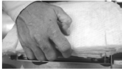
Figure 8 Remove Fiberglass Insulation
