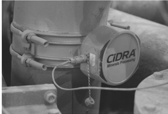
Figure 20: Sensor Head Assembly Mounted to Pipe
