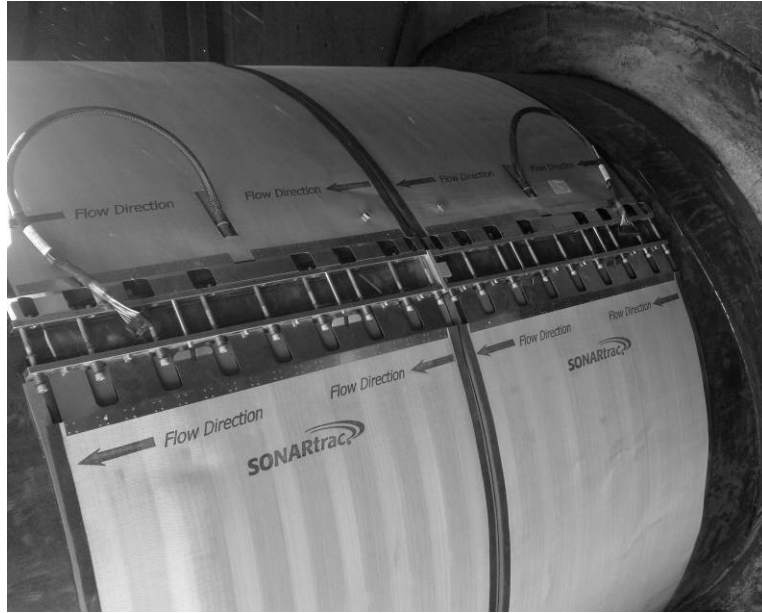
Figure 6 Sensor Bands Installed on Pipe
