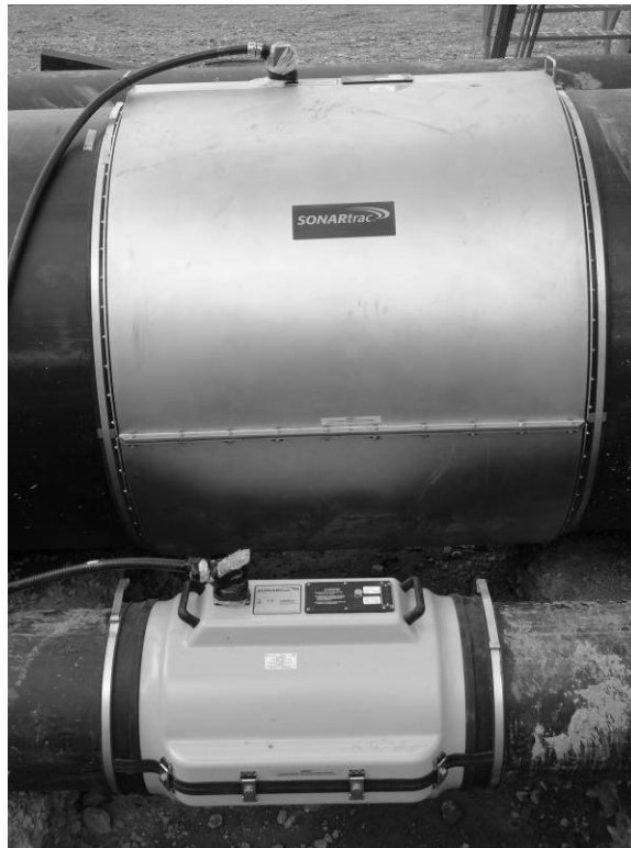
Figure 7 54" and 16" Installed Sensor Heads
