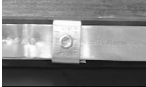
Figure 24 Boot Seal Wrapped Around Boot Seal in Groove
