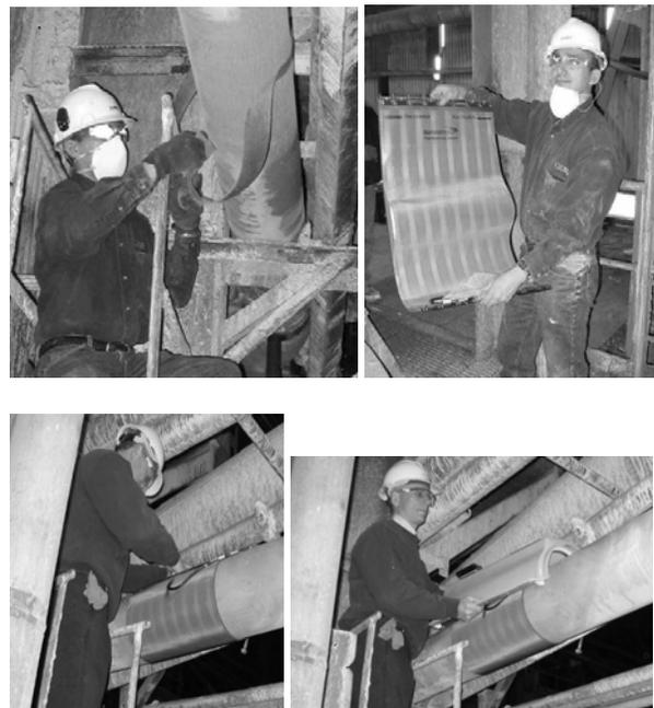
**Figure 4** Installation Procedure for Externally Mounted Gas Void Fraction Meter
